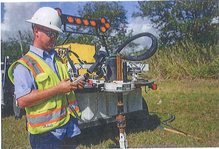
Valve operator Justin Wonsch exercises valves along a highway right-of-way.
